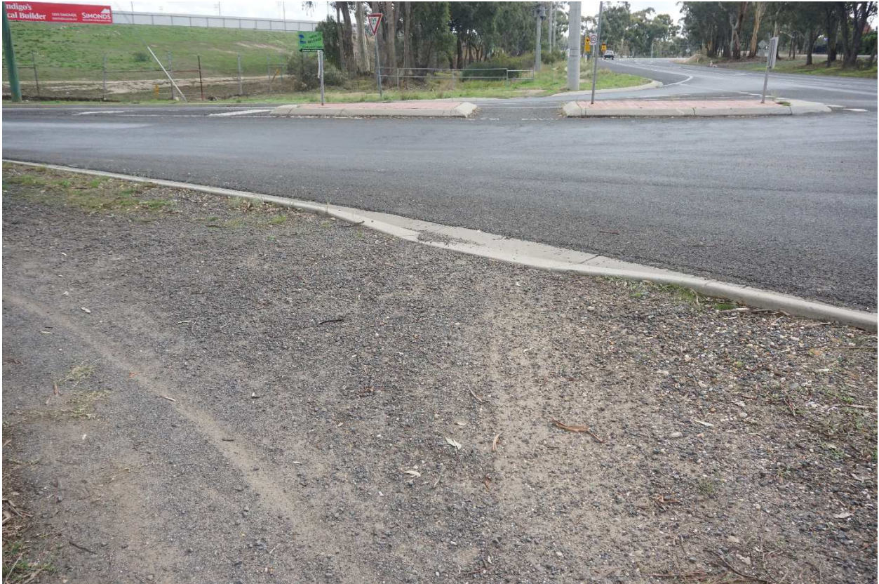
SECTION 3 – LOOKING WEST ACROSS ST VINCENTS ROAD
