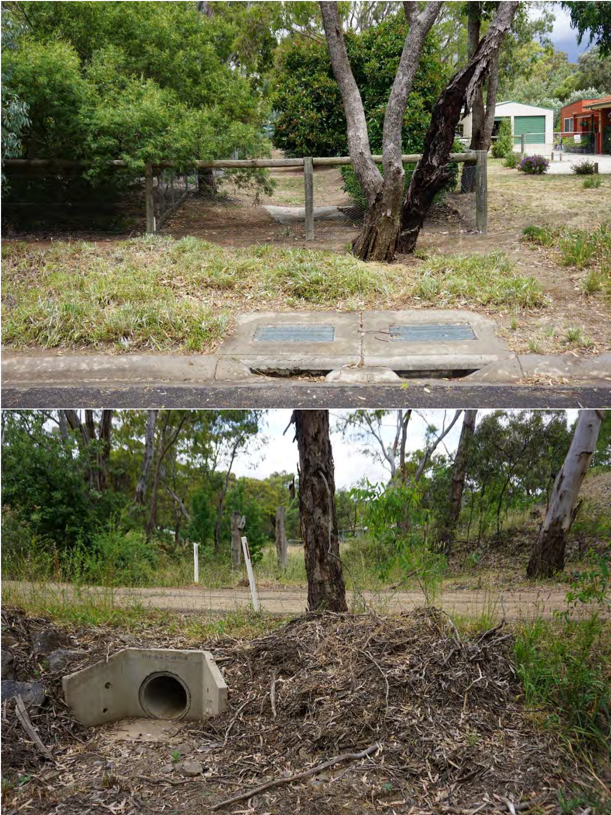
Figure 3-2 Upstream Overland Flow Path and Cleared Culvert
