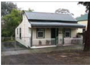
Typical miners' cottages with gable roof and rear skillion.
