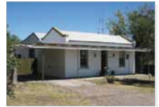
Double gable roof extensions, creating the distinctive zig-zag outline of a miner's cottage.
