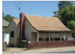
Double gable roof extensions, creating the distinctive zig-zag outline of a miner's cottage.
