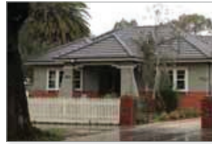
Roof cladding that has been replaced to match the original in form, pitch, colour and style.
