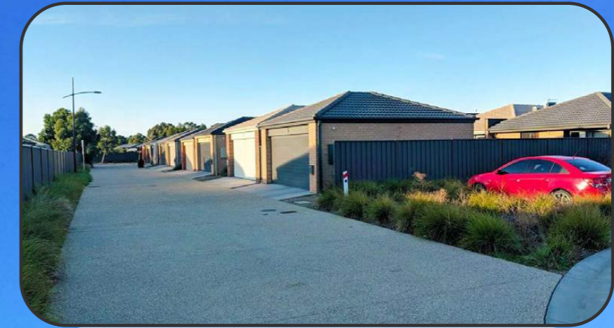
Rear access to the lots in the image below
