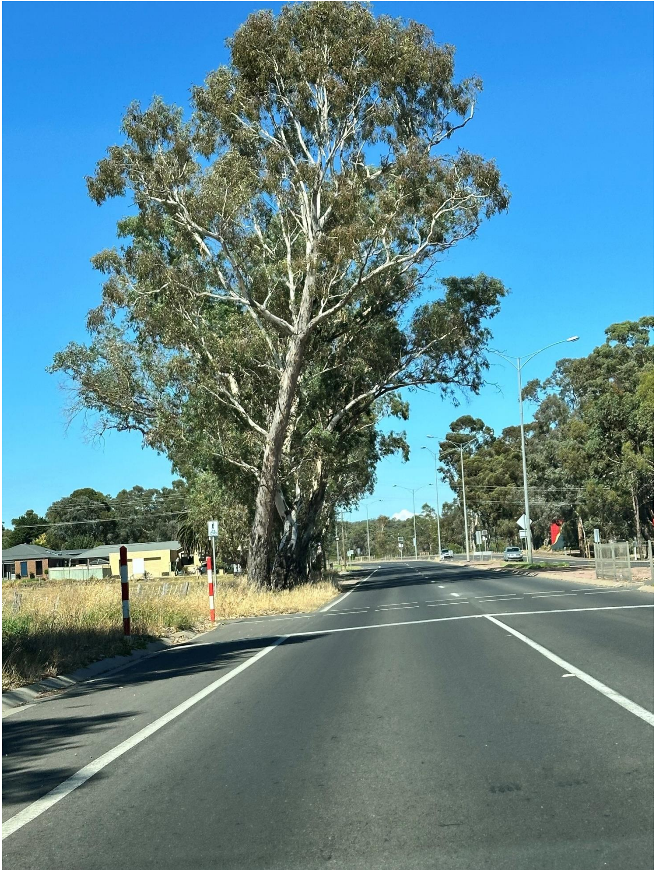
Figure 5. Looking south along Calder Highway towards the school crossing and intersection with Phillis Street (photo taken Monday 18 March 2024, midday)
