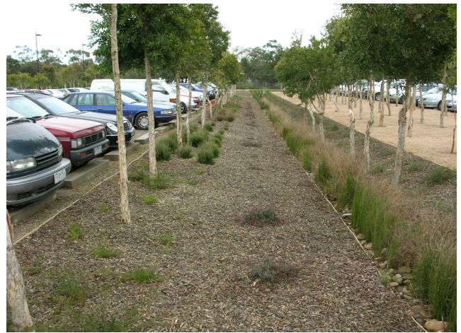
Figure 16. Locating a naturally vegetated swale within a car park increases visual amenity whilst providing passive infiltration
