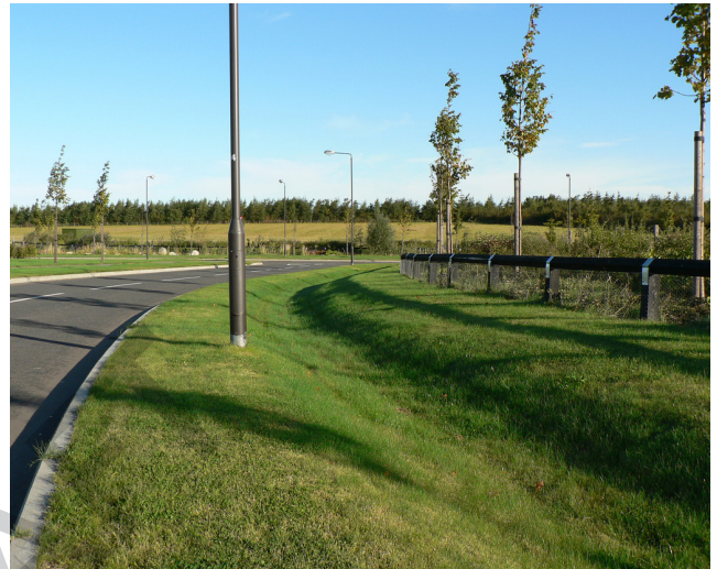
Figure 15. A grass channel incorporated into the road verge will passively treat storm-water run-off
