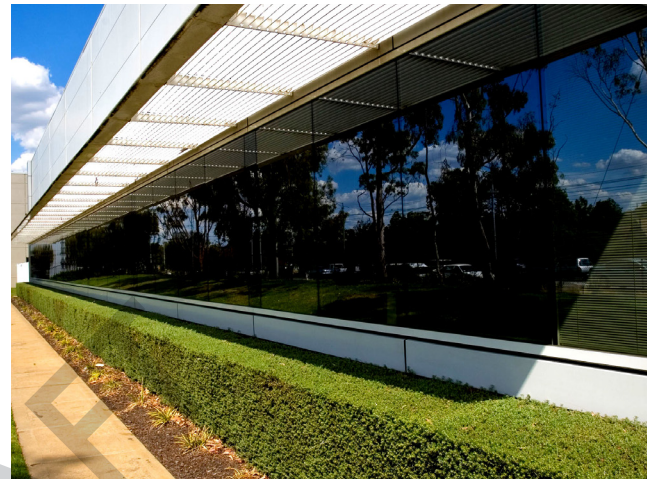
Figure 5. Fixed external shading devices are a simple and effective design element that reduce the heat transfer through the buildings fabric resulting in reduced energy demands
