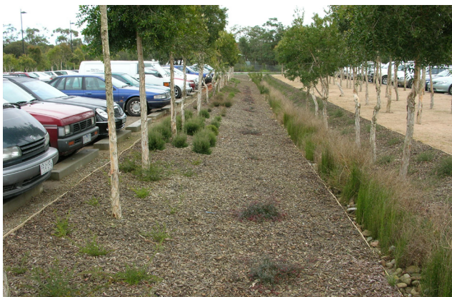
Figure 31. Example of a rain garden located within a car park to break up large areas of impervious parking areas
