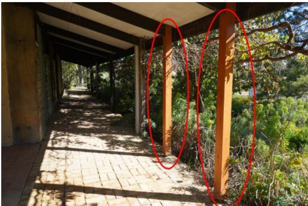
Figure 8. Verandah columns to be replaced
