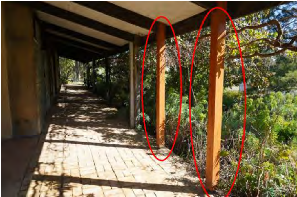
Figure 8. Verandah columns to be replaced
