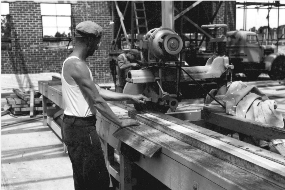
Figure 5 Bendigo mechanical plant constructing the prefabricated houses facing Mimosa Street, c1947-50 (SRWSC c1947-1962)
