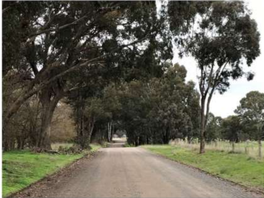
Photo 3: Looking south approaching floodway crossing
