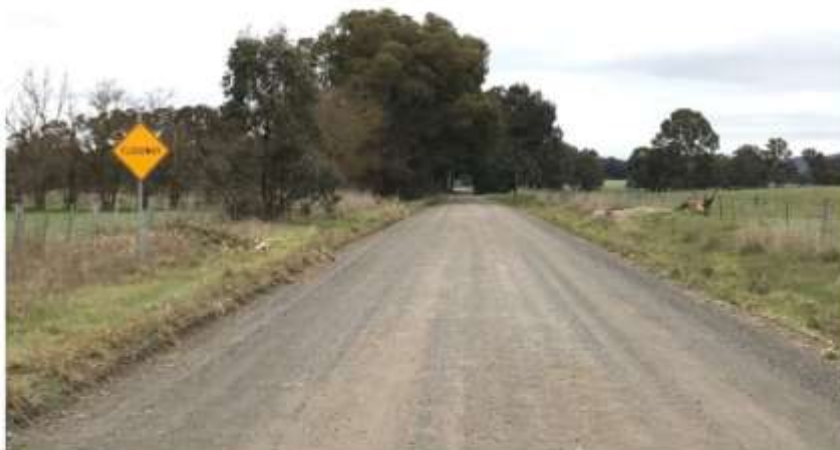
Photo 2: Looking south approaching floodway crossing
