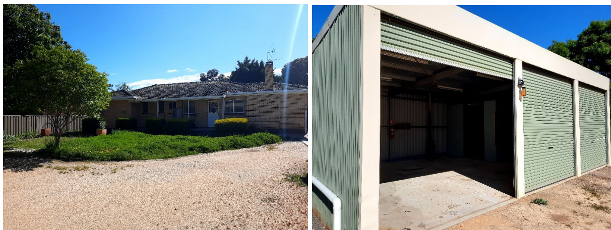
Figure 3: Rear of dwelling (proposed car parking location) and outbuilding (to be retained)
