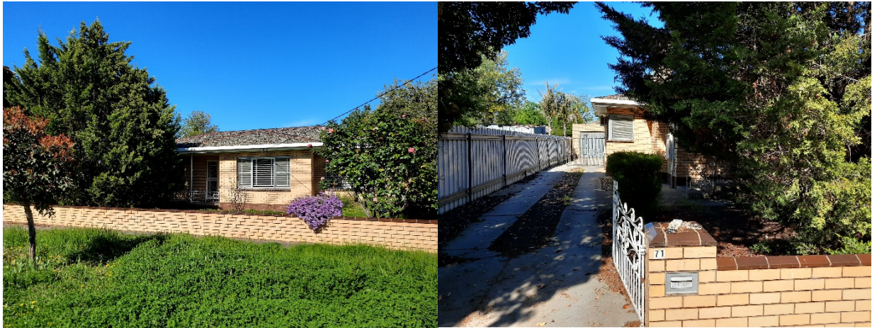
Figure 1: Photos of the existing dwelling
