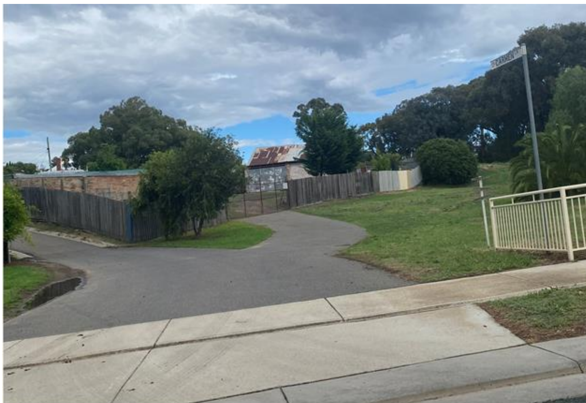
Figure 7: View of existing vehicle crossing from Ashley Street to Carmen Lane and rear of property at 10 Trotter Lane.
