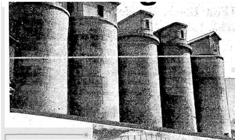
Figure 9. Five of the twelve concrete siloes at Darra constructed for the storage of cement, 1938, designed by John Beebe. (Source: Courier-Mail (Brisbane) 12 August 1938:9).
