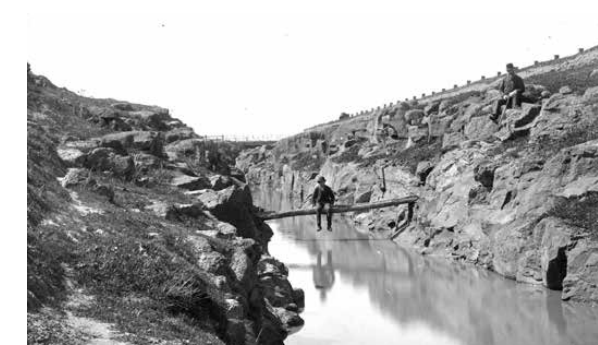
Bullock Creek channel diverting from the Loddon River c.1892 (source: State Library of Victoria)
