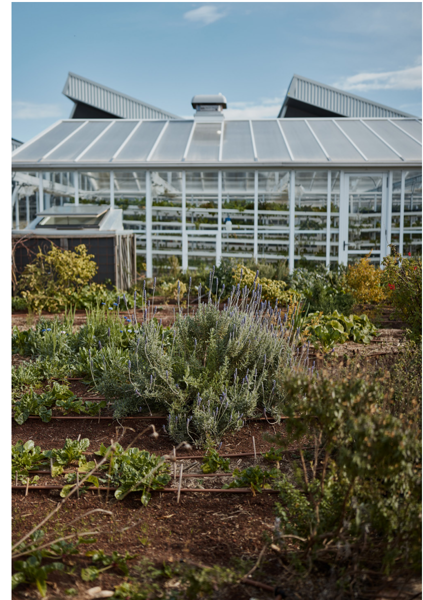
Rooftop garden and solar photovoltaic panels at Burwood Brickworks. Photography by Kim Landy
