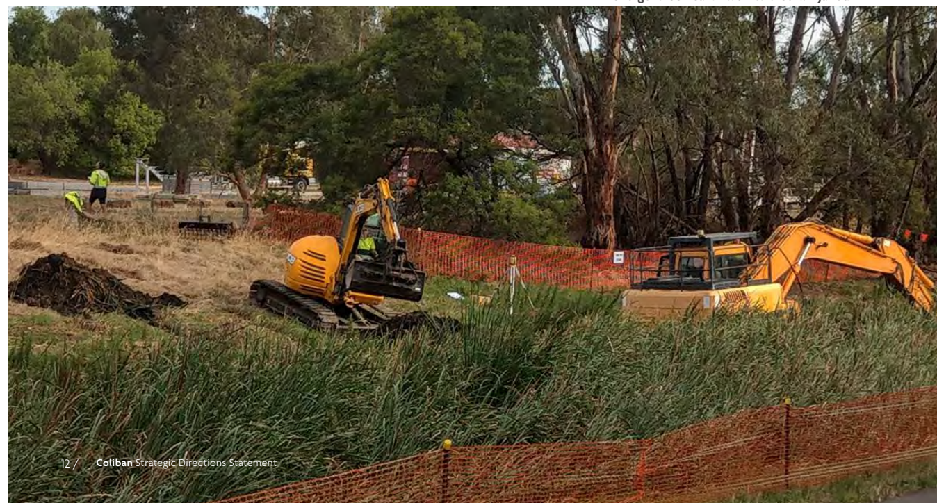
Bendigo Creek earth works. Credit: Djandak
