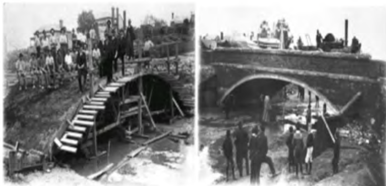
Turning the arch at Booth Street bridge (LHS) and testing the Booth Street bridge (RHS) c.1901. (Source: University of Melbourne Archives Image Collection cited in John Monash , nd)
