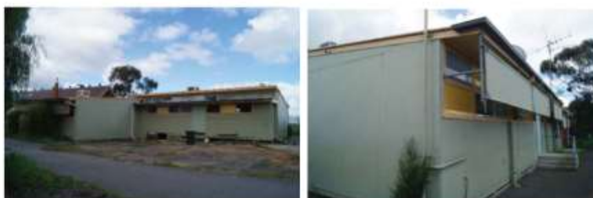
Examples of a cluster of Light Timber Construction (LTC) design units at Golden Square School since removed due to poor structural conditions and potential asbestos contamination.
