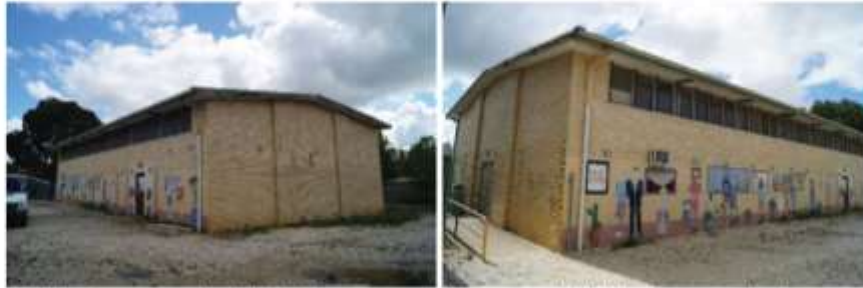
Hall simple rectangular light brick masonry wall structure with high clerestory windows.
